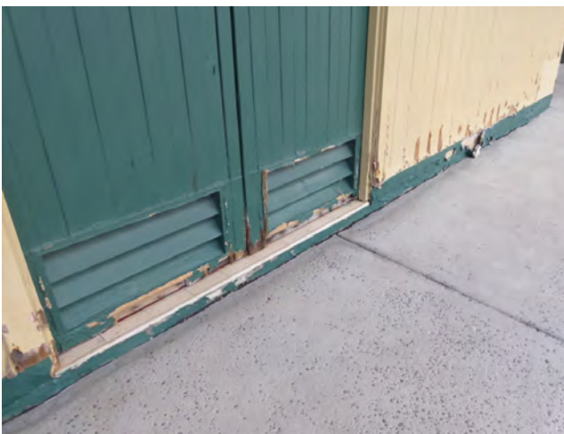
Figure 3.14 The timber near the ground floor walkway is rotting. This area is prone to flooding during king tides
