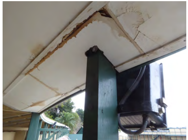
Figure 3.16 A water damaged ceiling sheet on the balcony of the 1926 Entry Building
