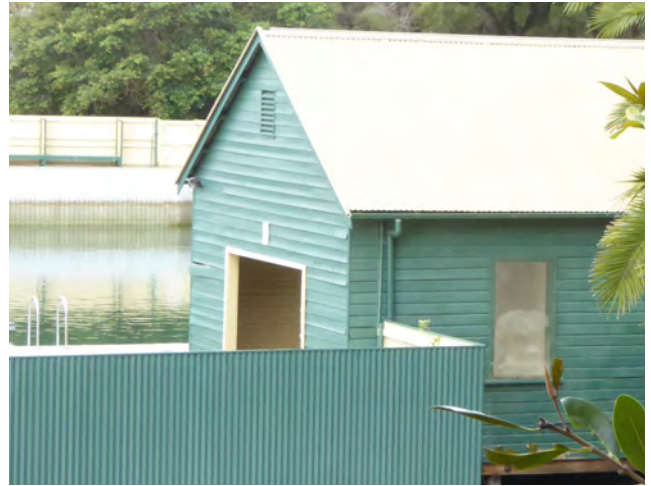
Figure 3.15 The cladding on the northern elevation to the Western Shed is distorted
