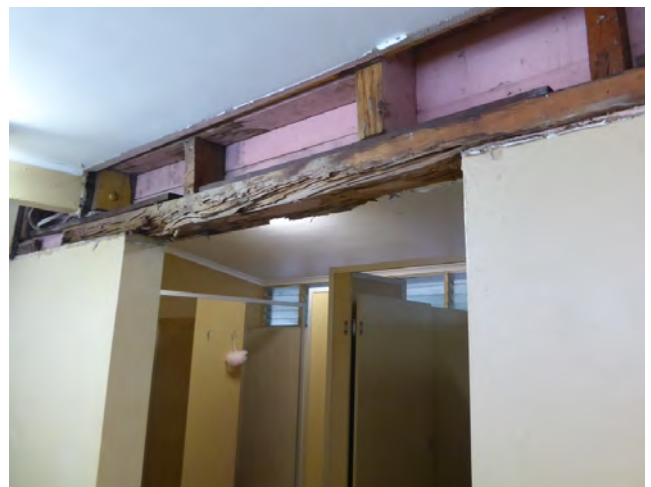
Figure 3.17 A highly deteriorated structural beam in the male bathrooms, on the line of the southern perimeter to the 1900 pavilion
