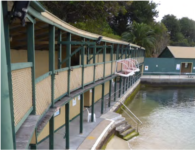
Figure 3.12 The roof line and first floor walkway are no longer straight but have twisted from exposure to the environment and aging
