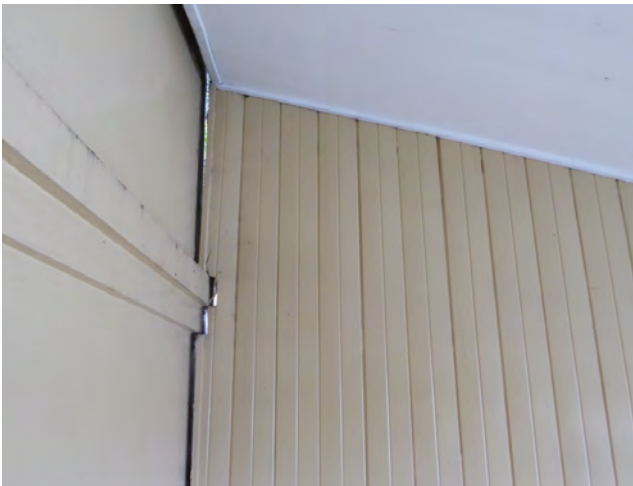
Figure 3.13 The end of the western side of the 1900 Southern Pavilion has pulled away from the masonry Entry Building
